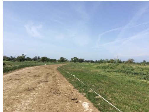
Figure 4: BMP#2 after, looking north.
