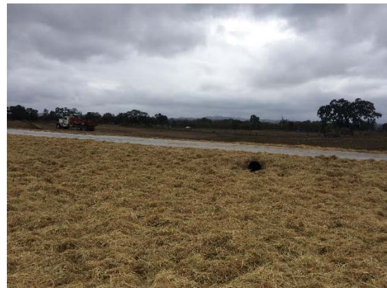
Figure 6: BMP#2 after, clean water crossing, looking west.
